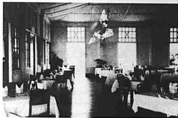
[Top and above] An outside view of the Crag Hotel and its dining room in the 1920s.
