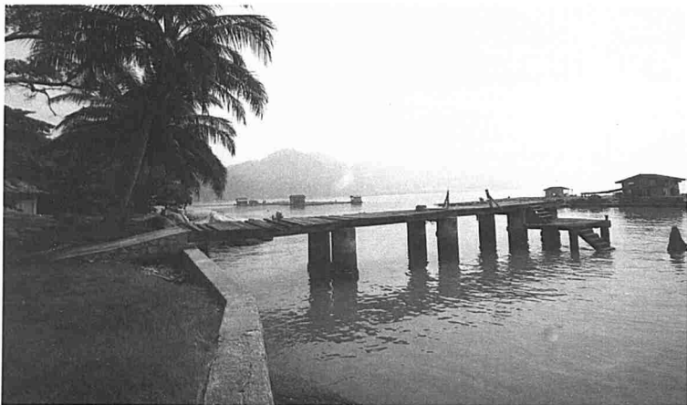
The old jetty still greets visitors to the old hospital and government quarters of Pulau Jerejak. [Opposite page top] Abandoned government quarters viewed from the sea, and one of the surviving hospital wards on the island.
